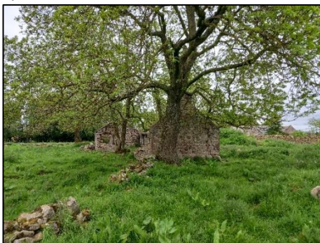
Photograph 5: Ruined building in the west of the site (proposed electrolysis plant area)
