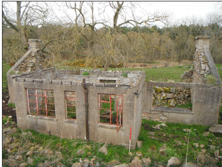
Figure 3.8: View facing north, providing an overview of derelict building remains which were part of the Dewsford farmstead (13).
