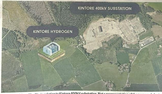
Approx. position of facility in relation to Kintore 400kV substation. Not a representation of the proposed plant.
